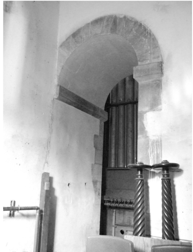
Fig 7. Photograph of north arch in central tower from the north; the wall on the left of the picture is the east wall of the north aisle (photograph: author).
