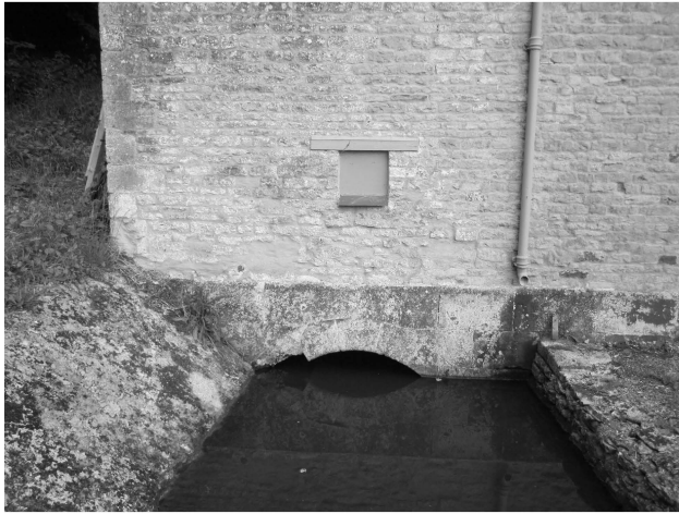
Fig 18. Tail race with sheepwash opening above.
